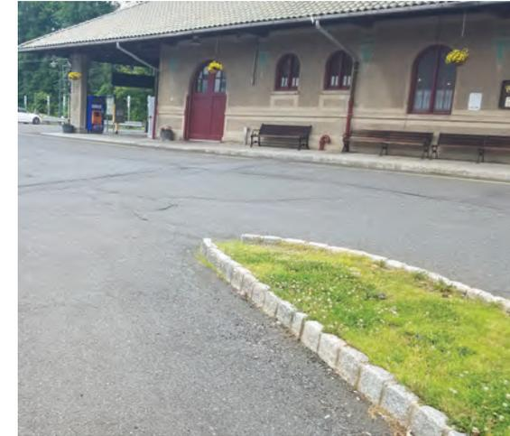
Downspouts on the north and south of the building can be disconnected and converted to planter boxes to capture stormwater runoff from the roof. Sections of parking spaces can be converted to porous pavement to capture and infiltrate stormwater runoff from the parking lot. A preliminary soil assessment suggests that more soil testing would be required before determining the soil's suitability for green infrastructure.
