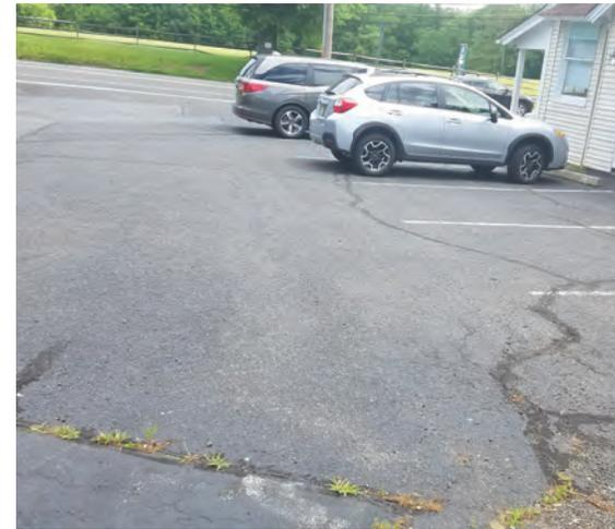
Parking spaces in the parking lot north of the building can be converted to porous pavement to capture and infiltrate stormwater runoff from the parking lot and roof. A downspout planter box can be installed under the downspout on the front of the building to help capture stormwater. A preliminary soil assessment suggests that the soils have suitable drainage characteristics for green infrastructure.
