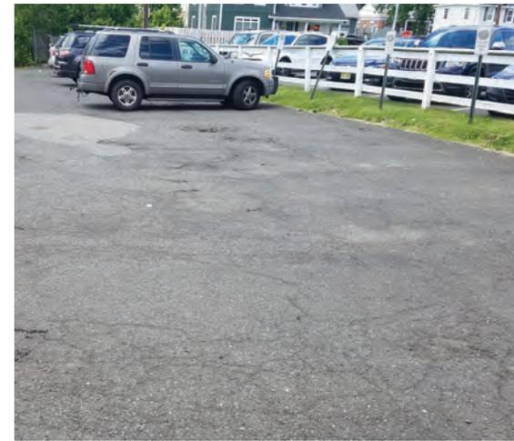
Parking spaces in the parking lot to the north of the building can be converted to porous pavement to capture and infiltrate stormwater runoff from the parking lot. On the north side of the building downspout planter boxes can be installed to help capture stormwater runoff from the building's roof. A preliminary soil assessment suggests that more soil testing would be required before determining the soil's suitability for green infrastructure.
