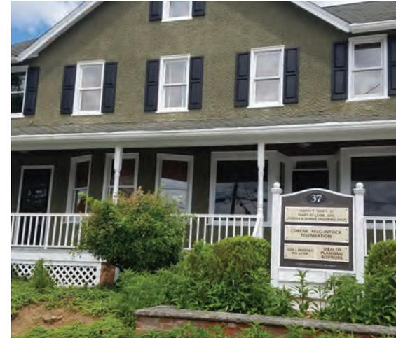
Downspouts on the northwest and southeast corners of the building can be disconnected and converted to planter boxes to capture stormwater runoff from the roof. A preliminary soil assessment suggests that more soil testing would be required before determining the soil's suitability for green infrastructure.
